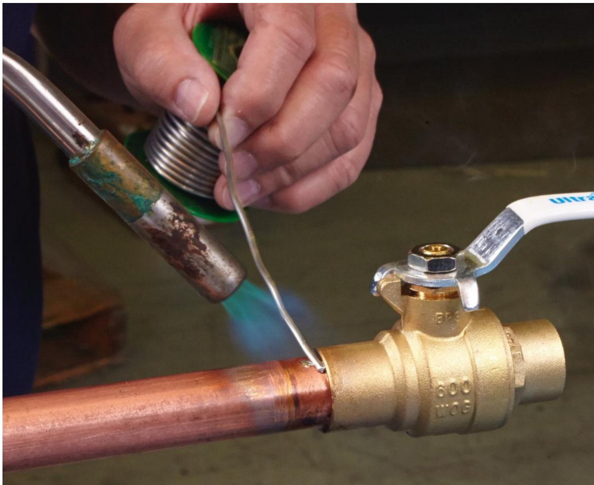
Milwaukee Valve UltraPure Ball Valve being soldered into a system.
