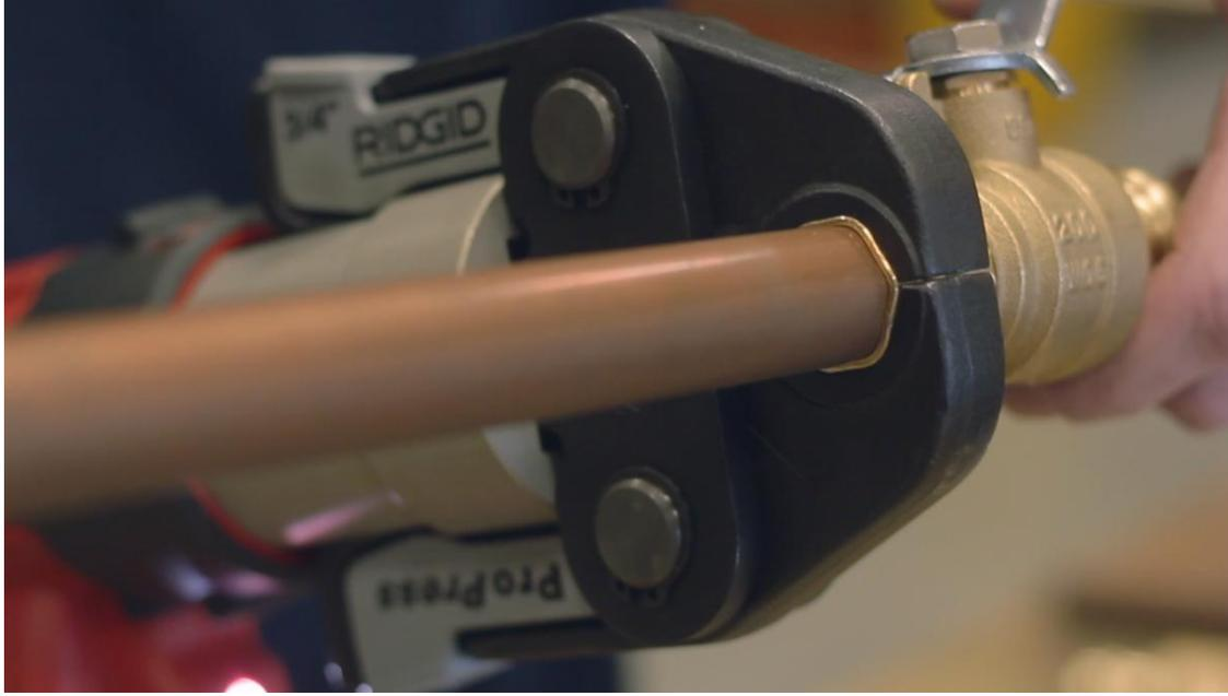
While some joint preparation is required (cutting and deburring), UltraPress valves substantially reduce overall installation time — up to 68%. That's the equivalent of three UltraPress valves installed in the same time period as one soldered valve.
