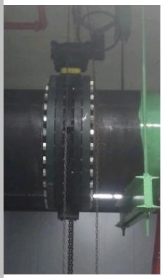
On the other hand, note this installation with a 36" resilient-seated valve. When using such large valves, it's recommended that the stem be installed vertically. Having the valve upright minimizes any sideloading of the bearings and liner, due to the weight of the disc. This is only important in the larger diameter sizes.
