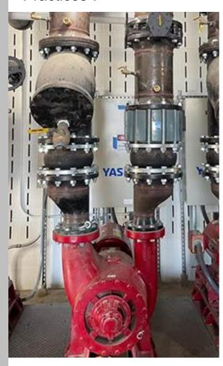
Recently, a report was received that several silent check valves were leaking in an installation. All were leaking at the mating flange. Upon further investigation, a few installation issues were uncovered.
