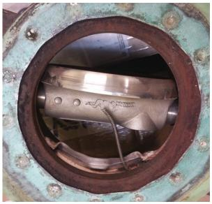
For best results and to avoid damage to the valve, HP throttling applications should be limited to 50 psi and the disc should be in between 30 and 70 degrees open. Due to the characteristics of steam, if a disc is positioned less than 30 degrees open, it creates high velocity flow in the area between the disc and the seat. This high velocity steam can pull part of the seat out, which gets crinkled
