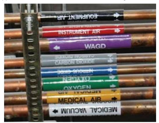
But what are these medical gases and what are their primary uses? Below is a list of the most common gases found in many healthcare facilities. These gases can be delivered and stored in cylinders or tanks on-site, or larger facilities may even have their own air separation plants on site and actually make their own.
