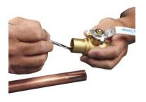
(4) Apply flux to the inside of cup of valve and outside of tubing. All surfaces should be covered with sufficient flux so that adhesion is assured. Do not use fluxes with contain ammonia or ammonia bearing compounds.
