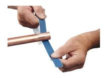
(2) The end of the tubing to be inserted into the valve cup should be cleaned to a bright finish, with steel wool, cleaning brush, or emery cloth.
