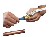
(3) The solder cup of the valve should be cleaned to a bright finish with steel wool, cleaning brush, or emery cloth.
